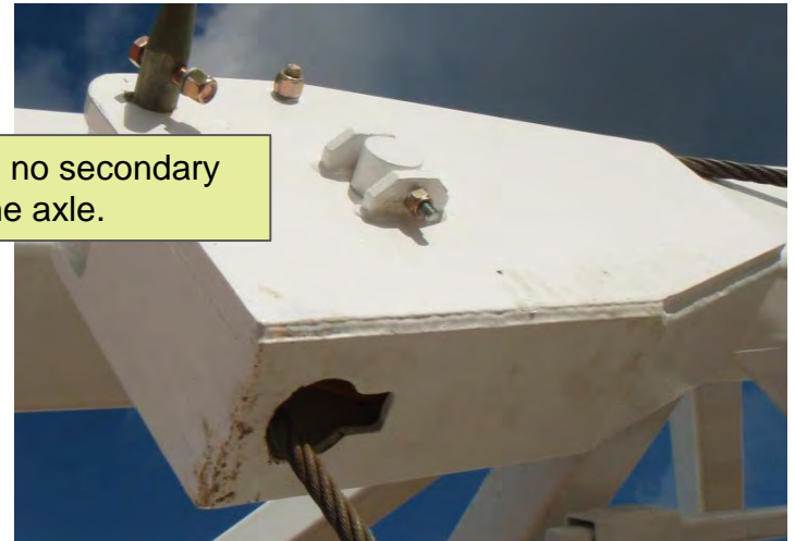
Crown mounted jib. Sheave secured to jib, but single pin hinge to mast.
