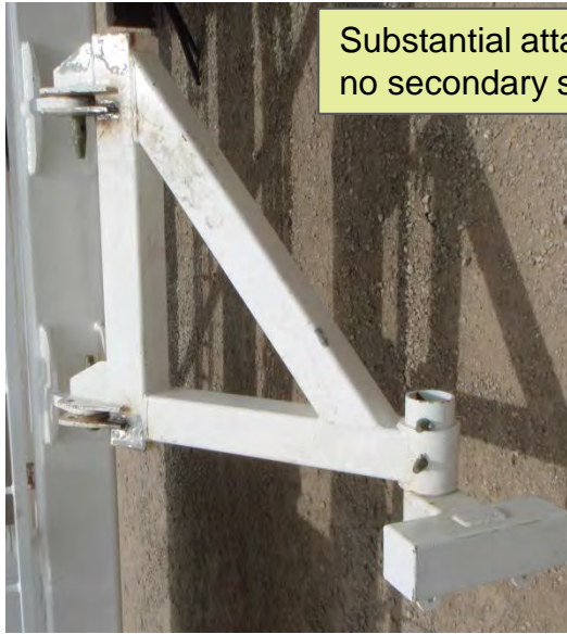
Brackets relying on securing pins.
