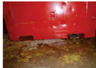
Holes for fork lift with the metal pieces within
