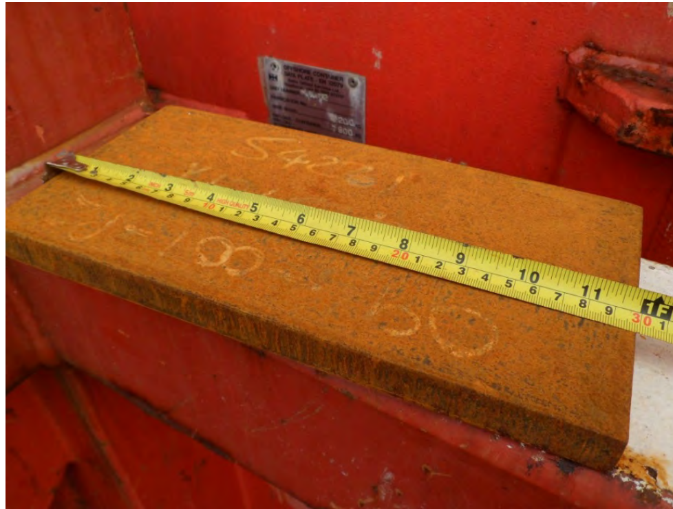
Piece of plate steel on the top edge of a unit
