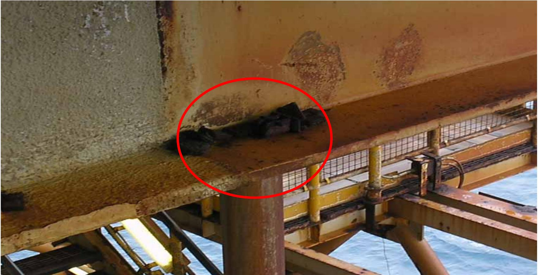
Redundant clamps left on beam – Unsecured Drops Hazard
