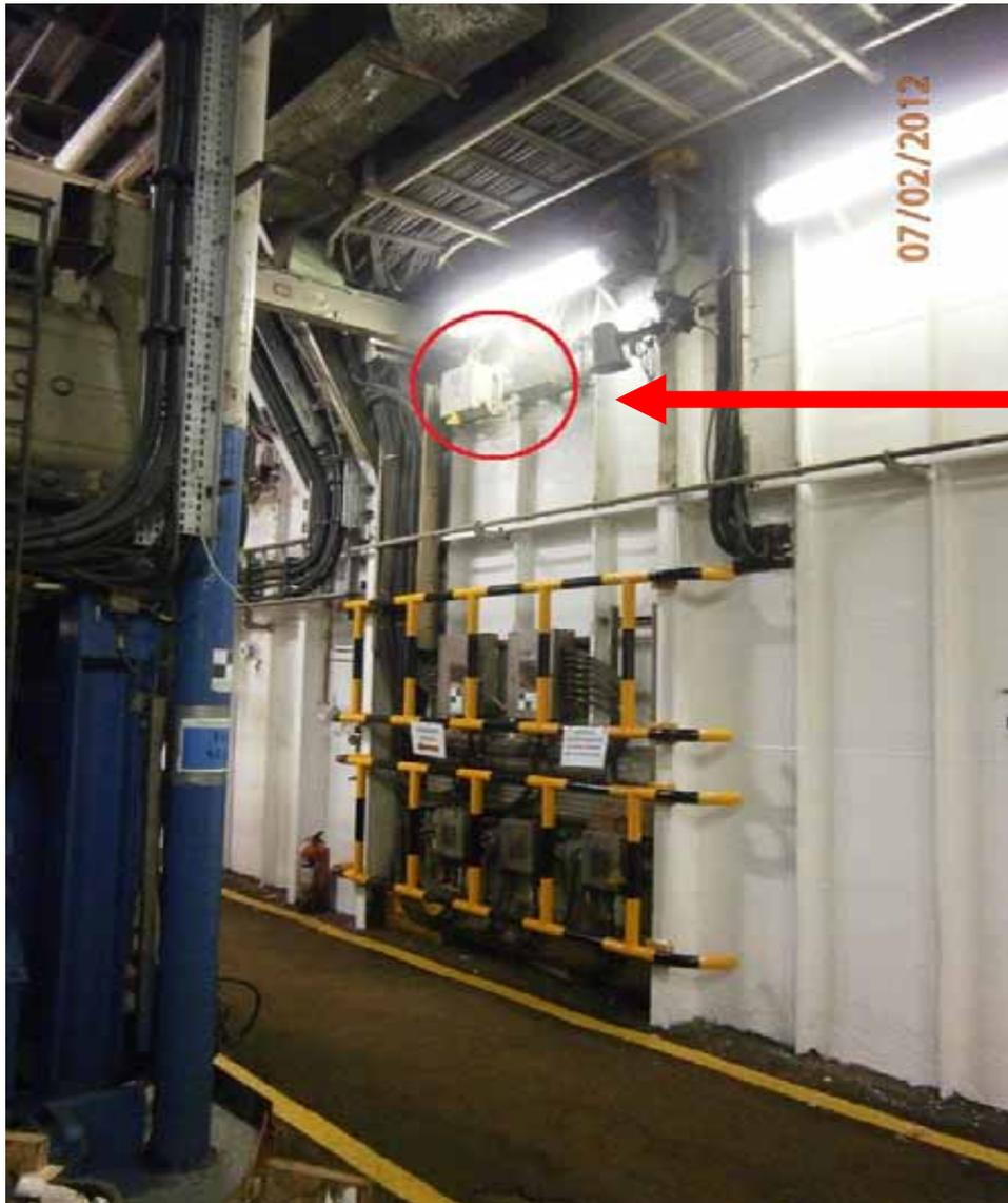
Two junction redundant junction boxes. Cables are still installed and boxes secured to unistrut. Boxes are approx 15 feet from the deck.
