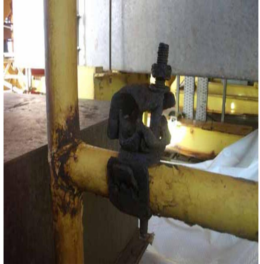
**A redundant handrail and scaffolding clamp left in place for some time.**
