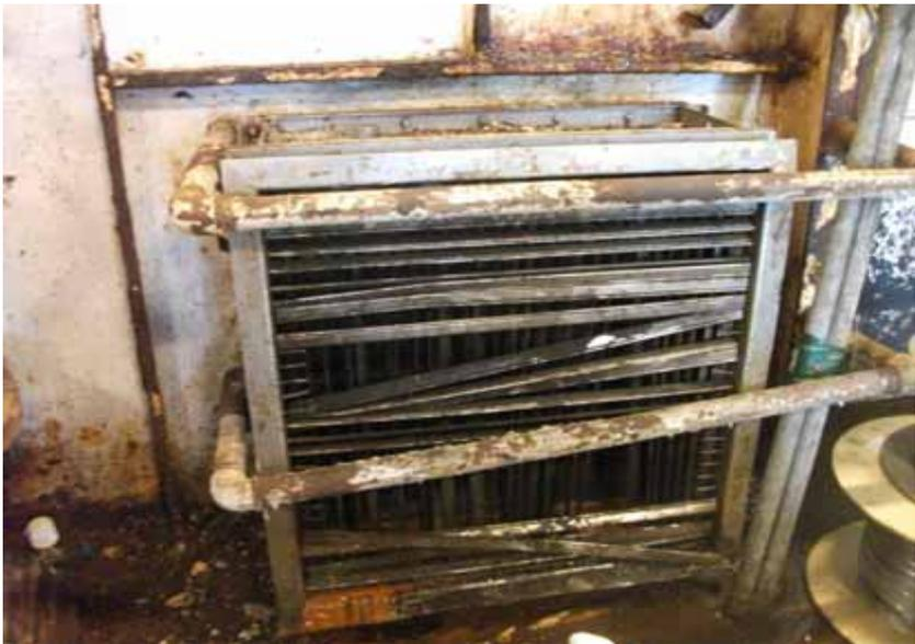
Redundant heat exchangers & HVAC units in the sack store.
