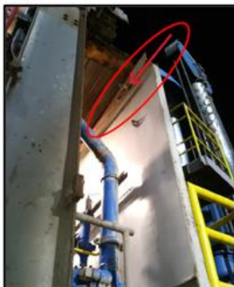
Figure 1. Drill Floor Deluge Line
