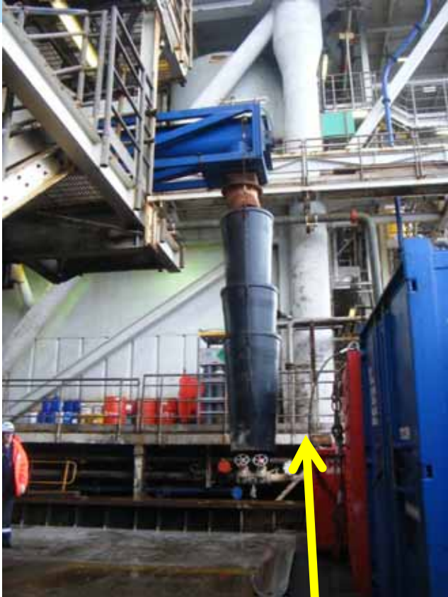
Cuttings chute in place (Dropped object removed)
