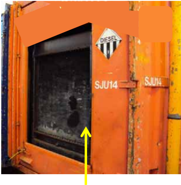
Unit on platform, following detachment of louver end plate
