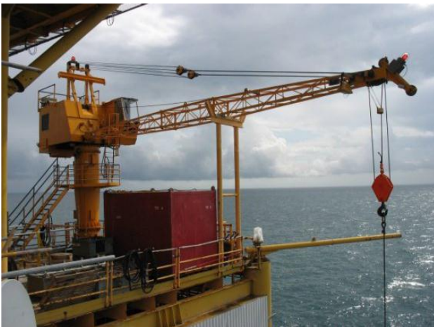
Crane before incident
