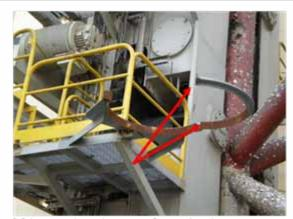
Make sure riser clamps on forward and port jacking structures are closed and bolts and nuts are tight.
