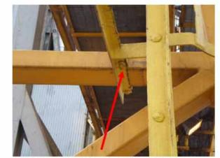
Check all bolts and nuts on the ladder for the Catwalk Machine.
