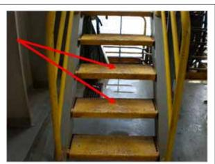
Check antislip stair treads on all stairs on cantilever are properly fastened.
