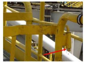
Check all gate bars on all levels have safety pins inserted.
