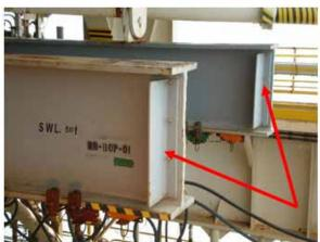
Check all end stops on both BOP runway beams are in place and properly secured.
