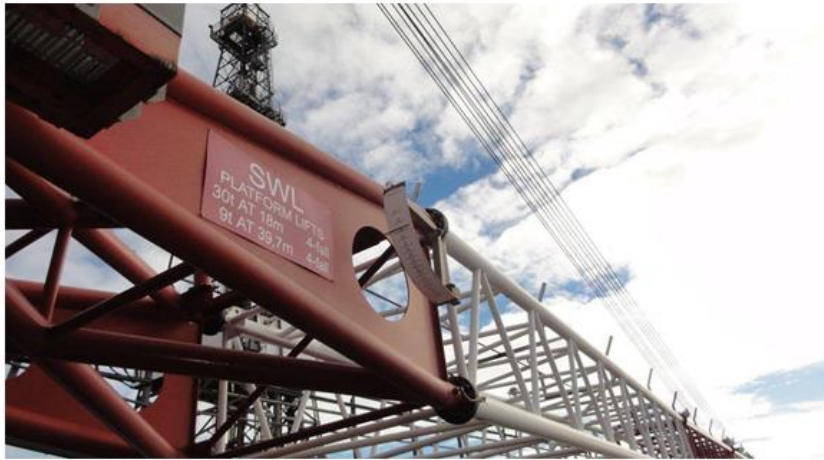
Inclinometer in position on West Crane, for reference
