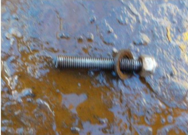
Sheared screwed rod as found on Pipe Deck
