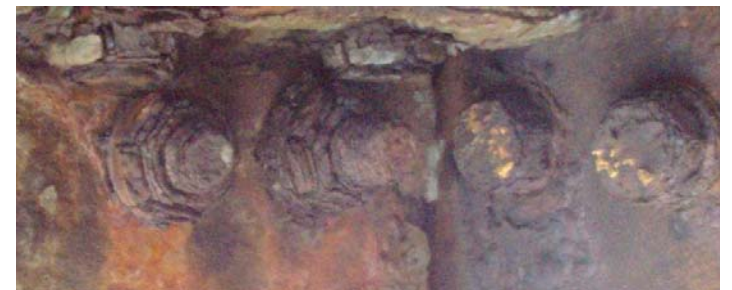
Corroded beam and saddles
